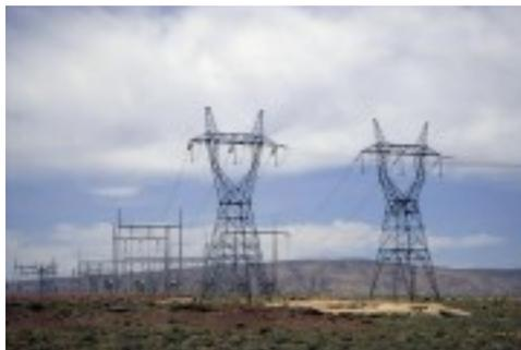
Voltages above 230 kV are considered “extra high voltage” and require different designs compared to equipment used at lower voltages. Overhead transmission lines are un-insulated wire, so design of these lines requires minimum clearances to be observed to maintain safety.(Wikipedia, Electric power transmission, 2007) See photo to the left and on the next page.
